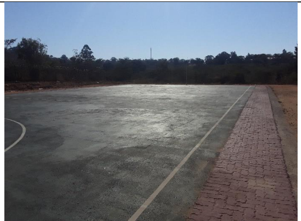
Fig.4.20: Netball Court in a satisfactory condition
