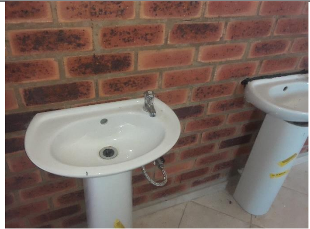
Fig.4.8: Silicone need to be applied on the sink
