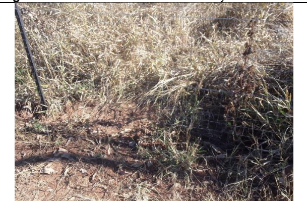
Fig.4.4: Fence to be tied to the poles to prevent any animals/people going underneath the fence
