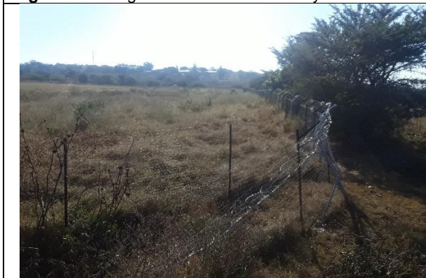
Fig.4.3: Fence on the southern border has collapsed/duplicated.
