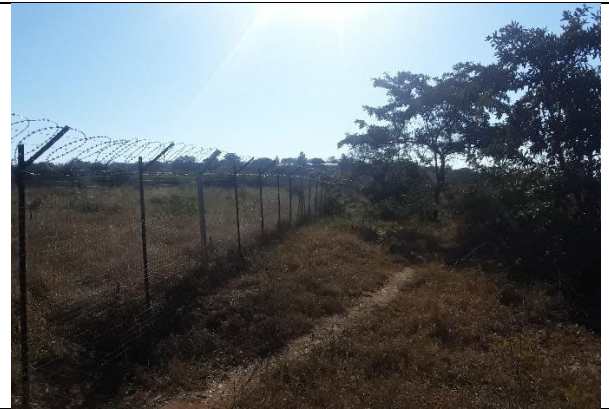
Fig.4.2: Fence is intact and in satisfactory condition
