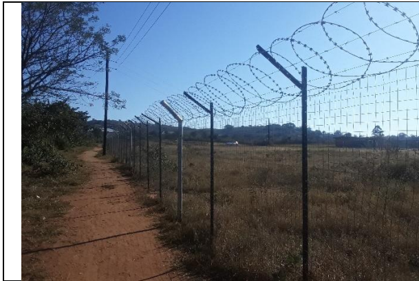
Fig.4.1: Fencing intact and in satisfactory condition
