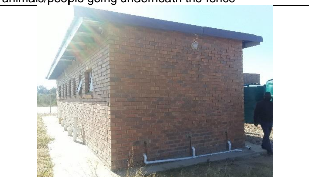
Fig. 4.6: Change Rooms in good condition
