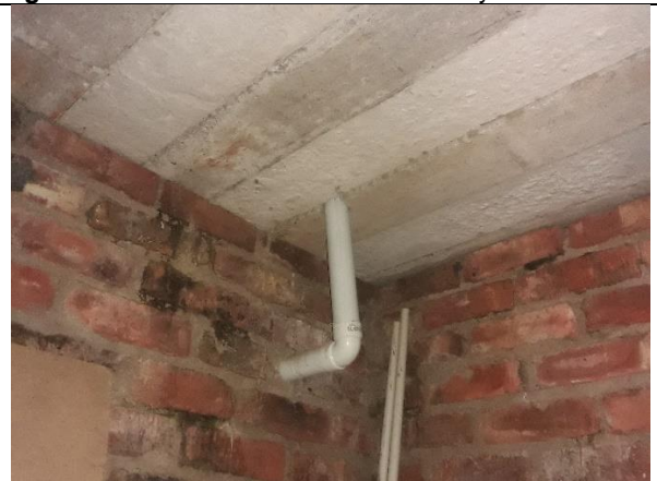
Fig.4.12: Storage Building Roof intact and in satisfactory condition
