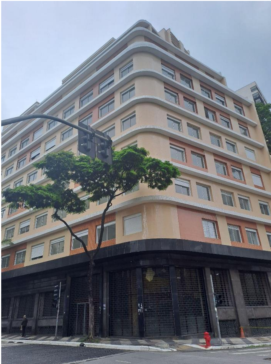
Elza Soares occupation after refurbishment. Source: authors; January 2023
