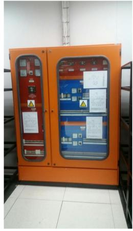
8.1302 The image below depicts the uninterruptable power supply (UPS) which comes into use immediately when a power outage occurs to bridge the gap in the power supply in the time the generator takes to start up. This ensures that there is a continuous supply of power to the datacentre.
